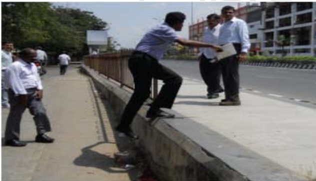
Figure 27: Excessive Heights of Footpaths Forces Pedestrians to Walk in the Carriageway.
