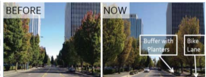
Figure 19: Portland, Before and After Installation of Protected Bike Lane Using Planters as a Buffer
