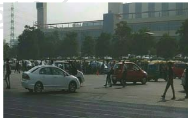
Figure 29: No Clear Demarcation for Pedestrian Road Crossing
