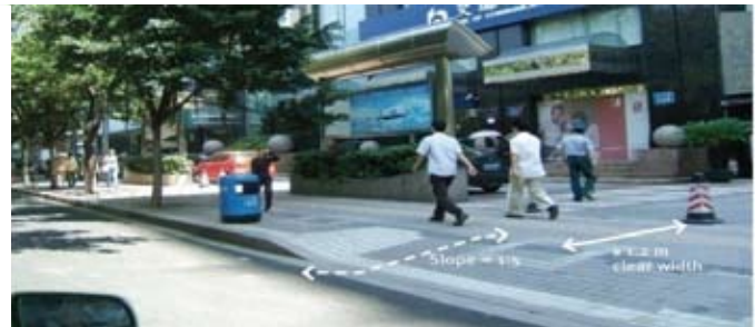
Figure 63: Curb Ramps and Footpaths with Tactile Paving
