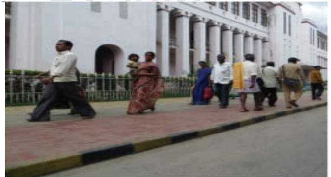
Figure 28: Footpaths with a Height of Not More than 150 mm are More Likely to be Used. 55
