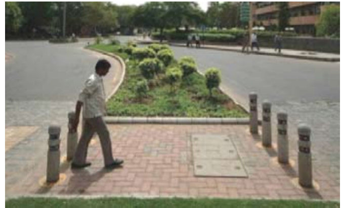
Figure 26: A Pedestrian Refuge Should be as Wide as the Crossing and Should Allow a High Volume of Pedestrians to Wait Before Crossing. 54
