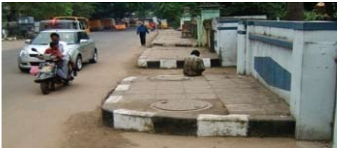
Figure 62: A Footpath that Constantly Changes Levels Discourages Disabled Pedestrians from Using it.
