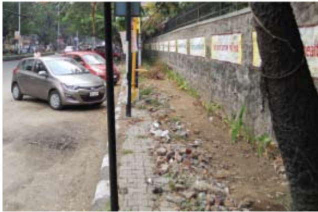
Figure 21: An Uneven Surface Can Make a Footpath Difficult to Use
