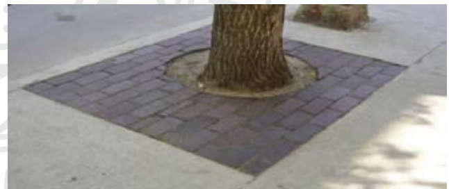
Figure 64: High Contrast Pavements around Planters and Other Obstructions if They are on the Sidewalk
