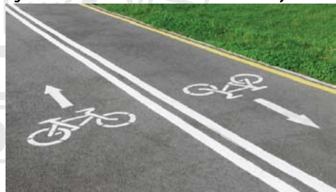
Figure 13: Exclusive Bicycle Path Adjacent to The Footpath 32
