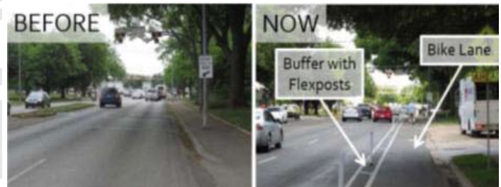
Figure 18: Austin, Texas, Before and After Installation of Protected Bike Lane Using Flex Posts
