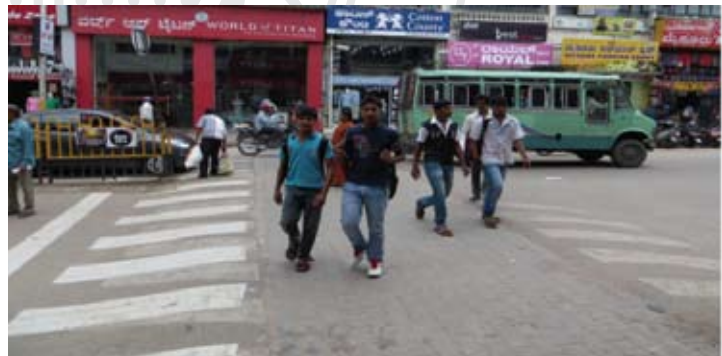
Figure 32: Raised Crossings Compel Vehicles to Reduce their Speed, thereby Increasing Pedestrian Safety. 57
